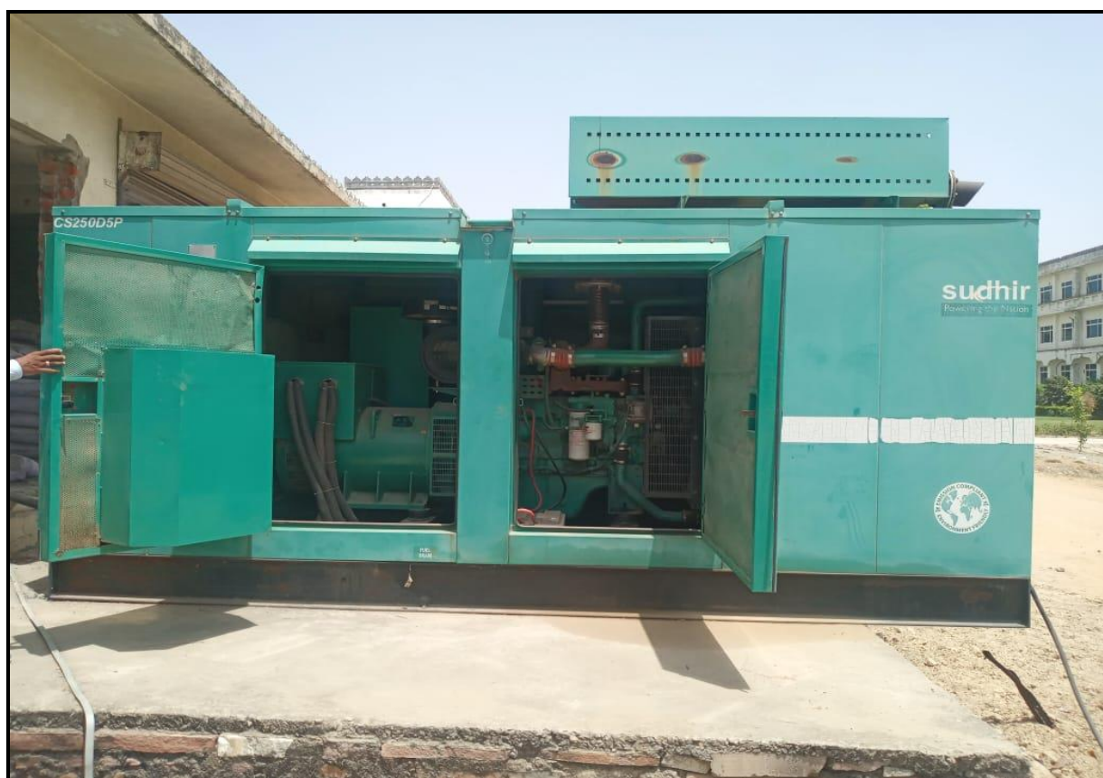
Figure 2.4:- DG set in Power House
