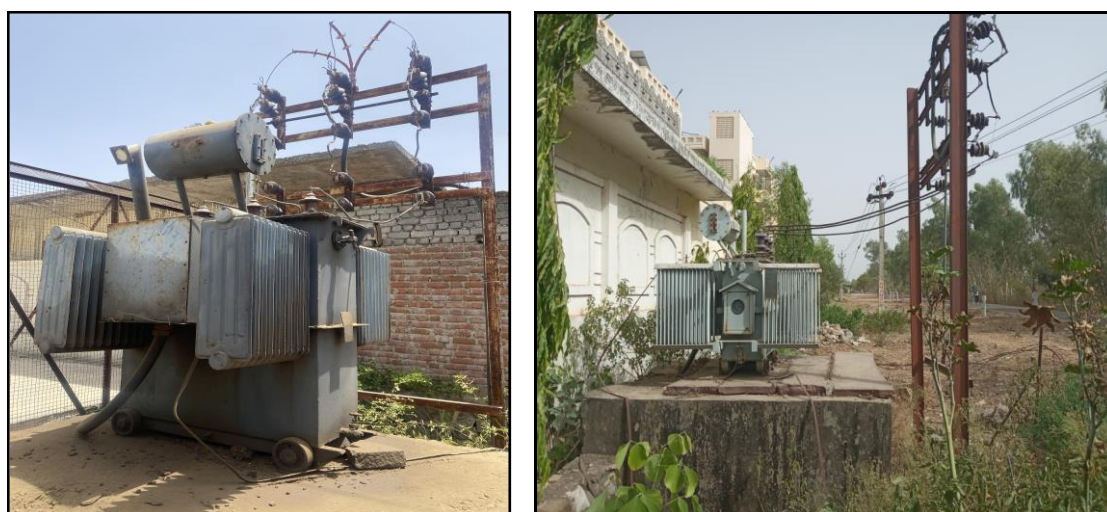
Figure 2.1:- 11 kV Feeder and 630 kVA and 500 kVA
