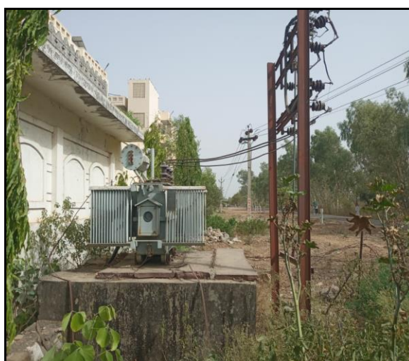
Figure 2.1:- 11 kV Feeder and 630 kVA and 500 kVA
