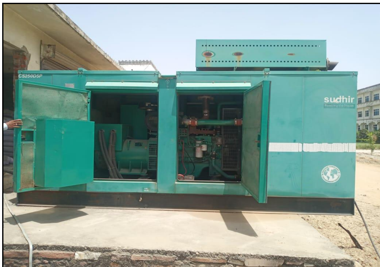
Figure 2.4:- DG set in Power House
