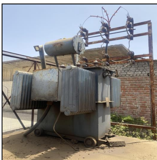
Figure 2.1:- 11 kV Feeder and 630 kVA and 500 kVA
