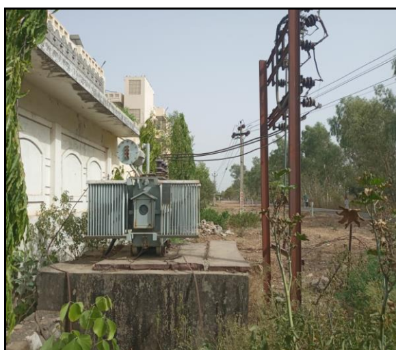
Figure 2.1:- 11 kV Feeder and 630 kVA and 500 kVA
