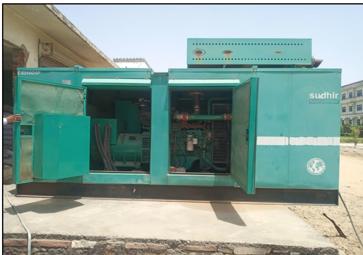
Figure 2.2:- DG set in the university
