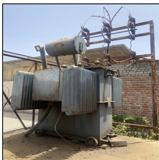
Figure 2.1:- 11 kV Feeder and 630 kVA and 500 kVA
