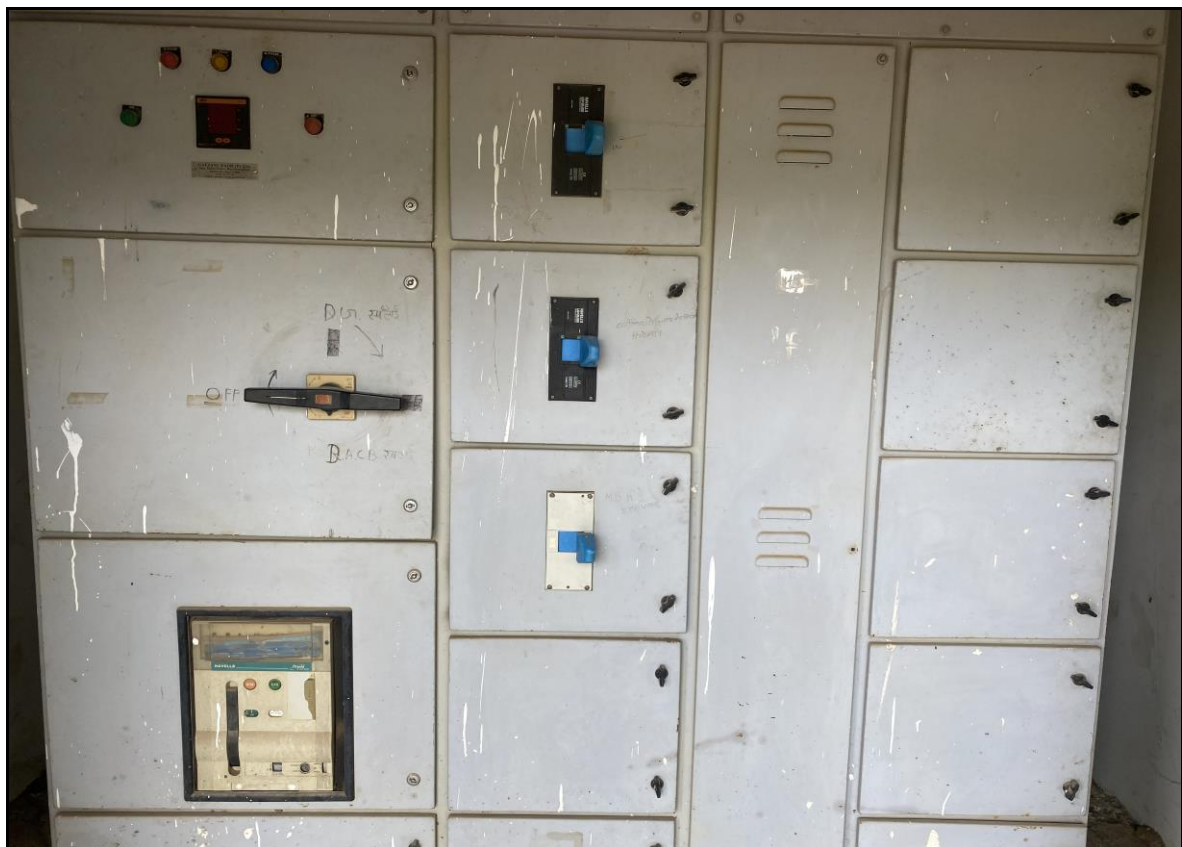
Figure 2.5 Capacitor bank on main panel
