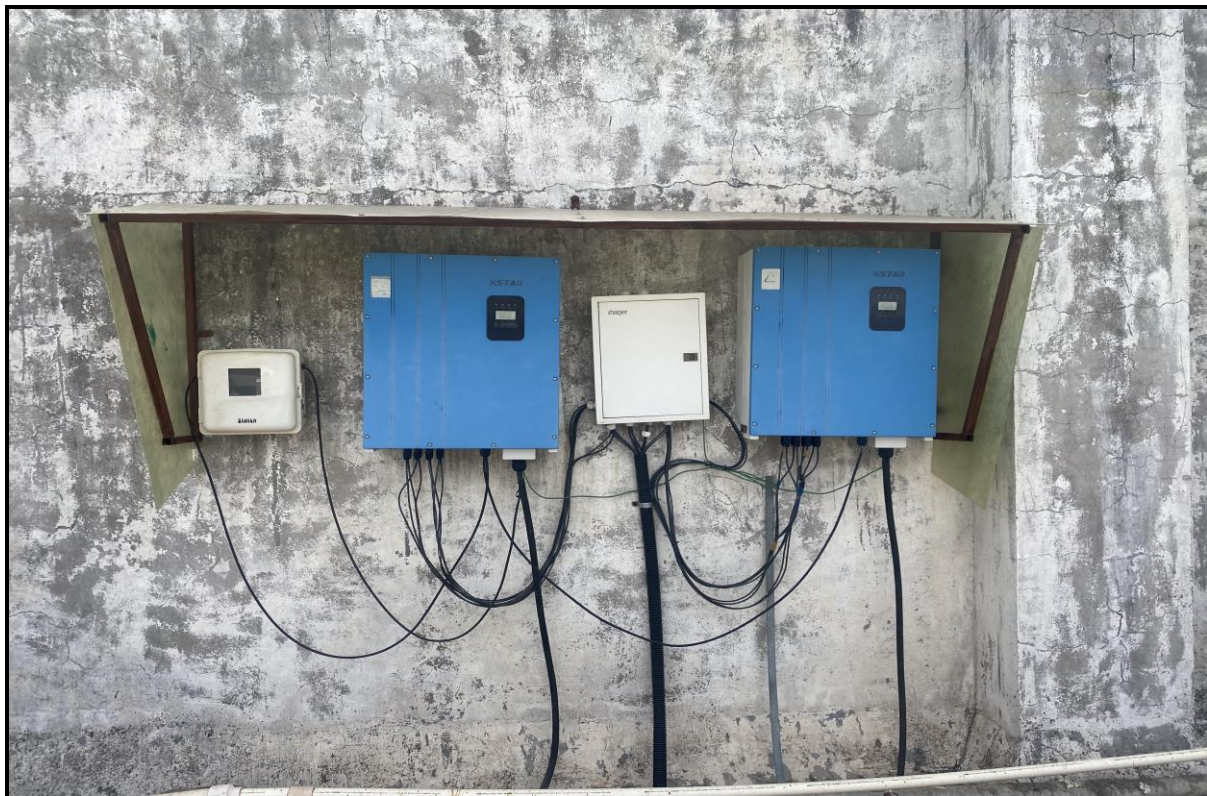
Figure 2.6:- Solar Plant 480 KWp and Inverter System
