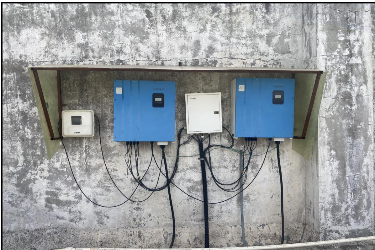
Figure 2.6:- Solar Plant 480 KWp and Inverter System
