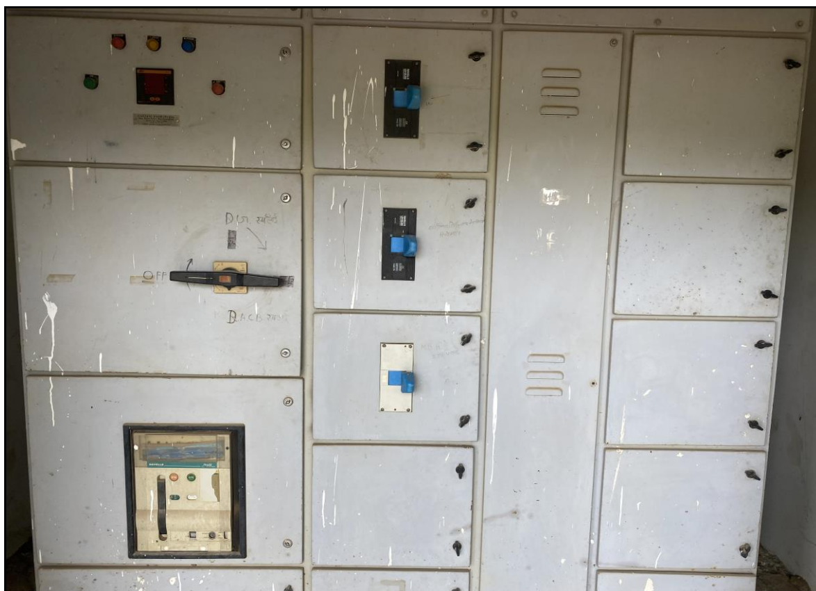
Figure 2.3 Capacitor bank on main panel
